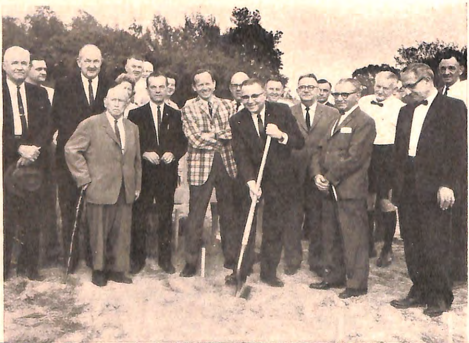
SUFFOLK, Virginia, Elks watch with pleasure as P.E.R. B. M. Scott, State Vice-Pres., breaks ground for their $80,000 home.
