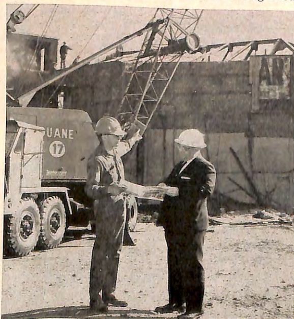
BRIGHTON, Massachusetts, Trustees Chairman Al Basse (right) is shown by engineer George Ross how demolition of an old theater building is progressing. The structure's unused portion was becoming a threat to passersby, so the lodge obtained an order to have the building razed.
