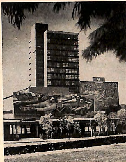
The University of Mexico campus has long been considered one of the most attractive and spacious on the continent. This is the administration building.
