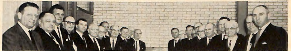
NEVADA, Missouri , Elks mark the completion of their new lodge building at a cornerstone-setting ceremony; E.R. Roy Brown (in group at right) presides. Visiting dignitaries included S.P. and P.D.D. William F. Gill, Kansas City, of Grandview-Hickman Mills Lodge; state Secy. G. K. McClintick, Kansas City, and D.D.G.E.R. R. Scott Roland and V.P. Galen Marr, both of Warrensburg. In the cornerstone capsule are lodge documents dating from the lodge's chartering. About 70 members and guests attended the ceremonies.
