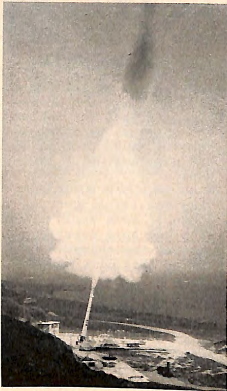
Though still experimental, Project HARP (High Altitude Research Project) already has sent rocket-boosted projectiles to 750,000 feet, conceivably could place small weather and communications satellites in Earth orbits at a fraction of the present cost. At the left is shown a spectacular firing of the 16-inch calibre, 119-foot gun (opposite page). The HARP installation on Barbados is diagramed above. Research is also being conducted to ascertain the feasibility of rocket-assisted artillery for Army use; an experimental, mobile 6-inch gun for this purpose is shown below.
