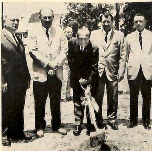
BRUNSWICK, Georgia, members celebrate the 66th anniversary of the granting of their charter by breaking ground for a new, $175,000 lodge building. PER and Judge A. A. Nathan, chairman of the building fund and a Trustee, turns the first spadeful of earth. Also pictured are Trustee A. P. Leotis and PERs and Trustees Jack Langford, A. Wright Knight, and Neal G. Gale. All have worked on the building program.
