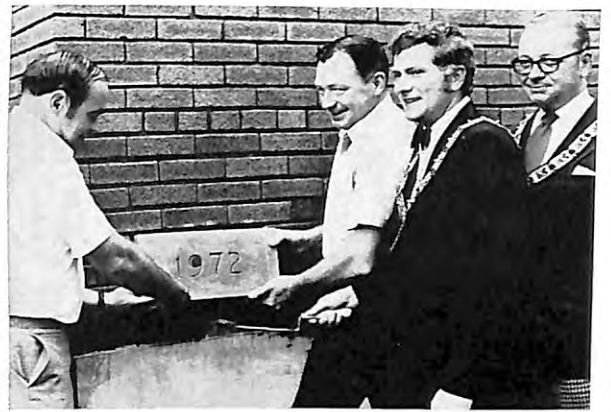
THE NEW HOME of Saratoga, N. Y., Elks was dedicated recently. Laying the cornerstone were (from left) building Chm. James Foley, construction Chm. Tom Fitzpatrick, ER D. Vaughn Woodworth, and dedication Chm. LeRoy Walbridge.
