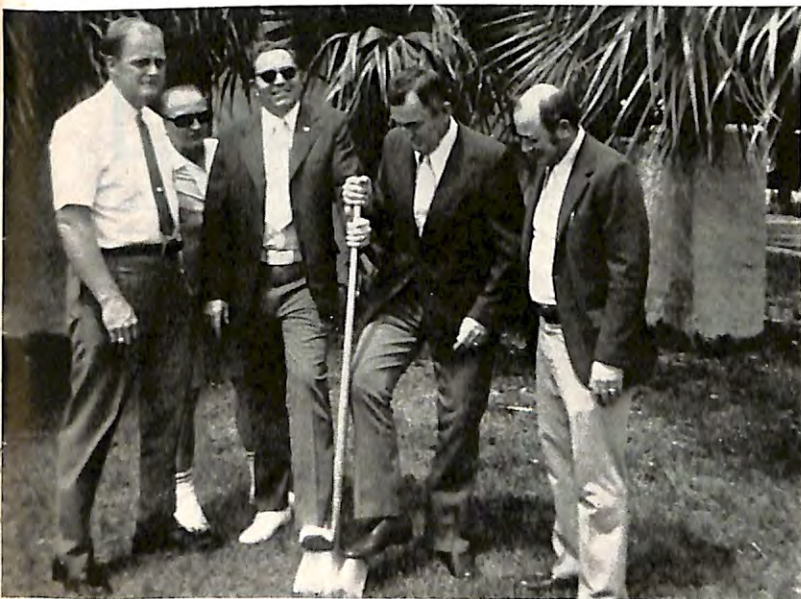
GROUND WAS BROKEN recently for the new home of Cocoa, Fla., Elks. Taking part in the ceremony were (from left) VP Frank Poitras Jr., PER Delbert Kreps, ER Charles Hunter, PER A. B. O'Hara, and Secy. Henry D'Amico.
