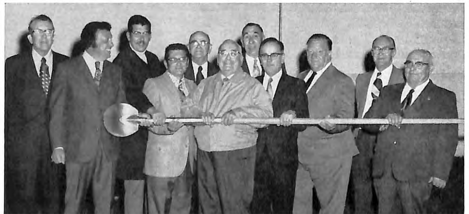
THE BUILDING COMMITTEE has been planning a new home for Boonville, N. Y., Lodge. At the ceremony marking the start of construction were (from left) Edward Sweeney, Felix Gaetano, Michael Golden, PER Louis Romeo, ER Howard Urtz, Secy. Fay Blum, Chm. Howard Gleasman, Louis Stocklosa, PER George Yocum, Harland Hayes, and Erwin Goodhines.
