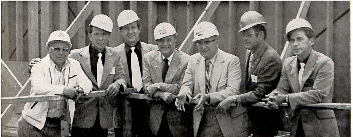
INSPECTING the site for the new home of Gateway, Ore., Lodge was then-GER Robert Yothers (center). With him were (from left) Al Schneibel, PER Richard Heath, PDD Tom Jones, PGER Frank Hise, SP Jim Damon, and ER Gene Pronovost.
