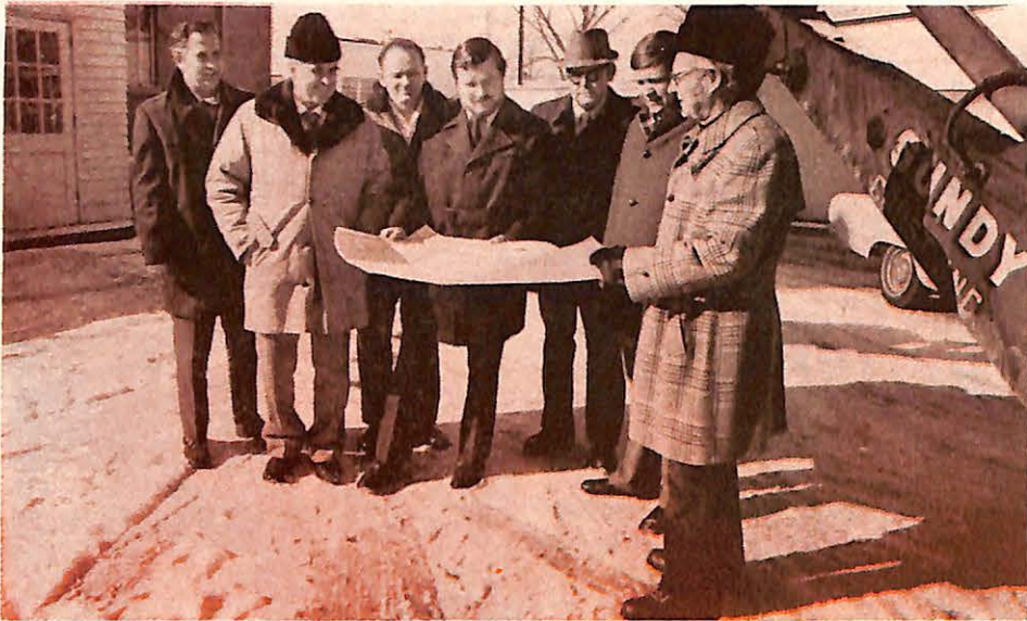
PLANS for a new addition to the lodge at Dover, Ohio, were studied by involved members at a recent groundbreaking ceremony. Contractor Ed Pongratz, Trustees Robert Ley and William Evans, Richard Fisher, architect, Trustee David Doutt, ER Richard Staley, and Building Committee Chm. Sherman Price were present for the event, which was the start of extensive physical improvements for the building.
