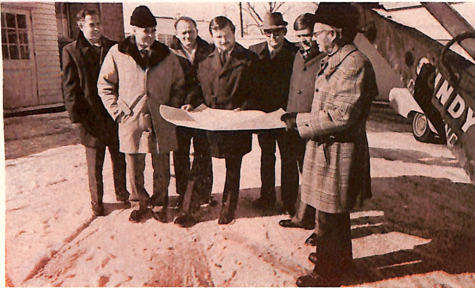
PLANS for a new addition to the lodge at Dover, Ohio, were studied by involved members at a recent groundbreaking ceremony. Contractor Ed Pongratz, Trustees Robert Ley and William Evans, Richard Fisher, architect, Trustee David Doutt, ER Richard Staley, and Building Committee Chm. Sherman Price were present for the event, which was the start of extensive physical improvements for the building.
