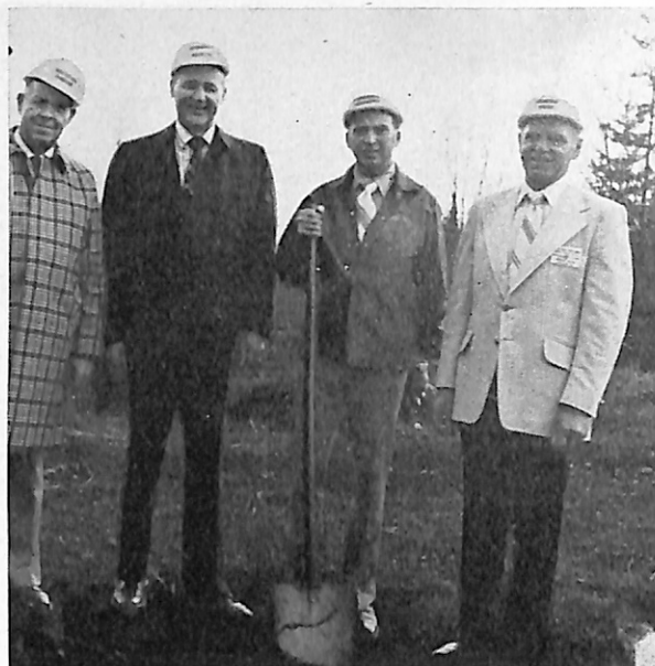
GROUND WAS BROKEN at Vancouver, Wash., Lodge recently for a new temple to replace the original building, which was constructed in 1910. Elks officers in attendance at the ceremony included (from left) VP Ivan Golden, SP Ted Butcher, ER Al Lighthart, and DDGER Dick Block.
