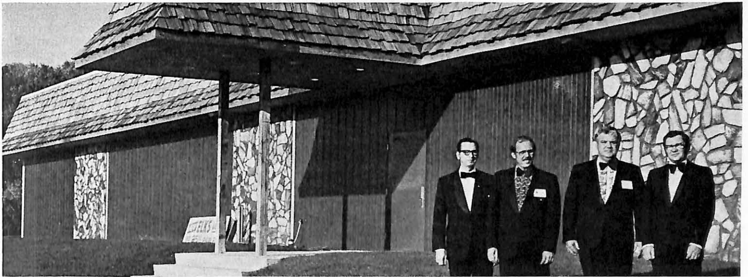
THE INSPECTION of Paw Paw, MI, Lodge's new building by (from left) DDGER Fred Tornquist, ER Fred Devantier, and PERs Dewayne Wiler and David Wilder was recorded by a Kalamazoo Gazette photographer during the dedication ceremonies. After the original lodge burned over a year ago, funds were raised for the erection of a new building, which the members completed themselves.
