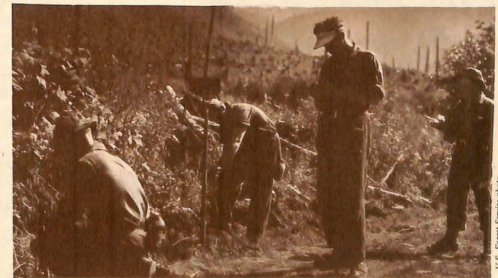
Surveying for a new road in Snoqualmie National Forest.
