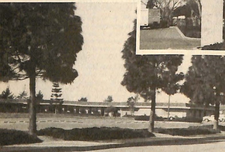
Low, modern architecture, spacious parking and an illuminated display welcome you to Elksdom's All-American Lodge.
