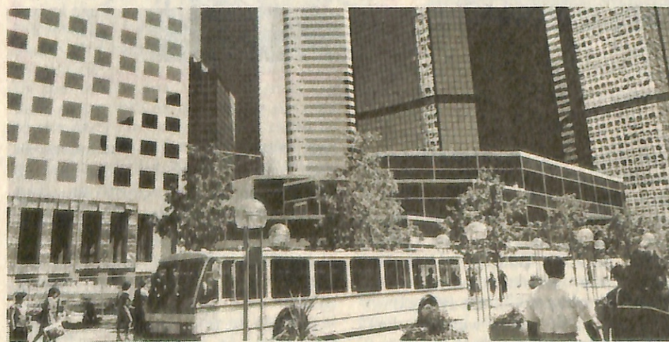
Denver's new $76-million 16th Street Mall stretches for a mile through the heart of the downtown business and shopping district.
