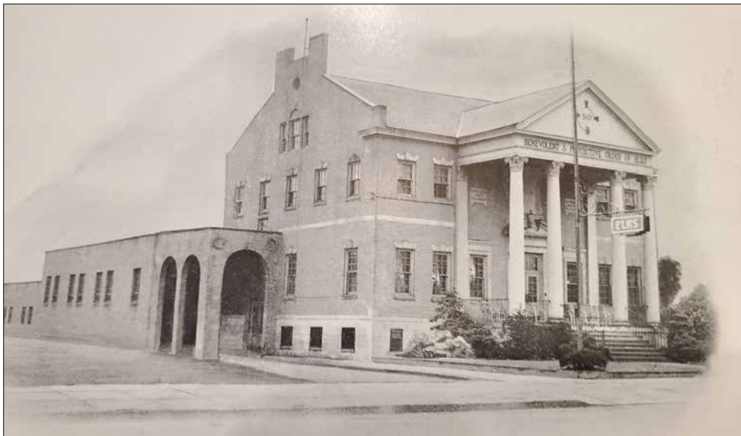
In the late 1940s, the New Philadelphia Elks #510 added a main bar, dining room, card room, ball room/back bar, and sauna/steam room. The project was dedicated in 1949 to coincide with the lodge's 50th anniversary. (Photo courtesy of Jeff Warner)
