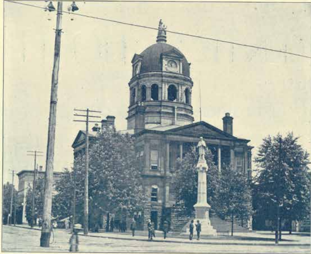
COURT HOUSE, NEW PHILADELPHIA, OHIO.
